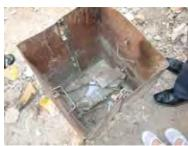
9. Backflow valve in access shaft.
