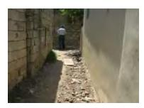
12. Compacted backfilled trench awaiting concrete pavement.
