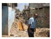
10. Newly installed pipes protected with course sand.
